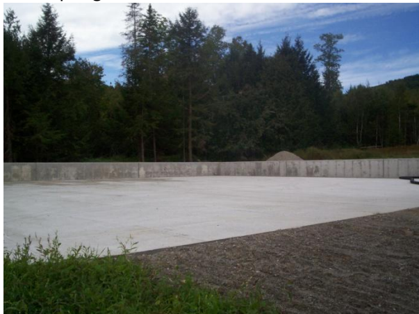
80' X 90' compost pad using 8' concrete blocks in 16' walls
